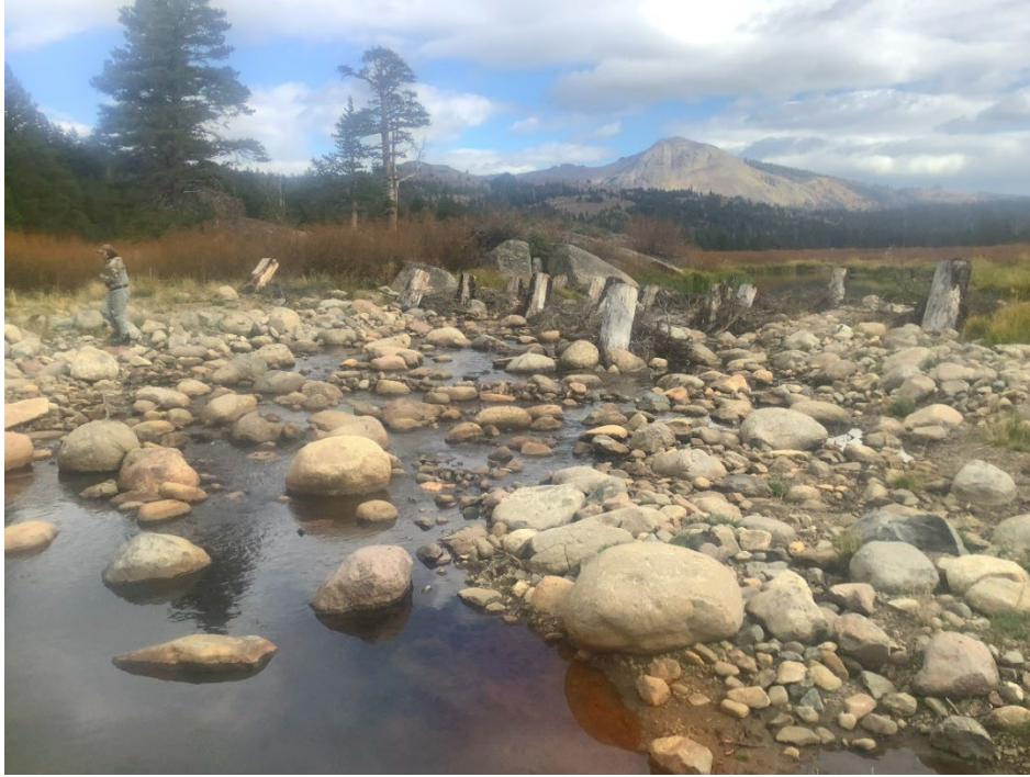
Figure 33. The grade control structure built at the downstream end of Faith Valley. The vertical logs coming out of the structure are intended to facilitate future beaver dams or beaver dam analogs by creating a sturdy anchor point. GM1_2024, FTRF1
