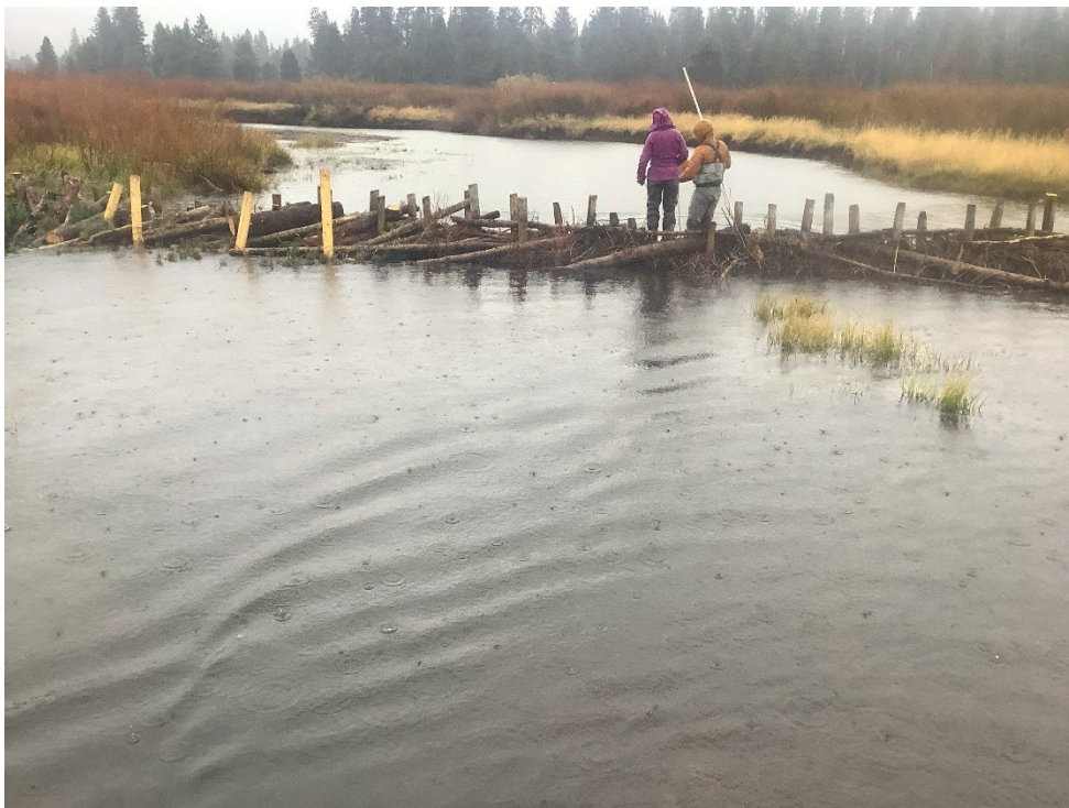
Figure 36. Just downstream of the previous photo in 2024 a BDA has been placed to aggrade the channel. The cutbank in figure 35 is visible in this image in the distance. GM1_2024 SDBV7
