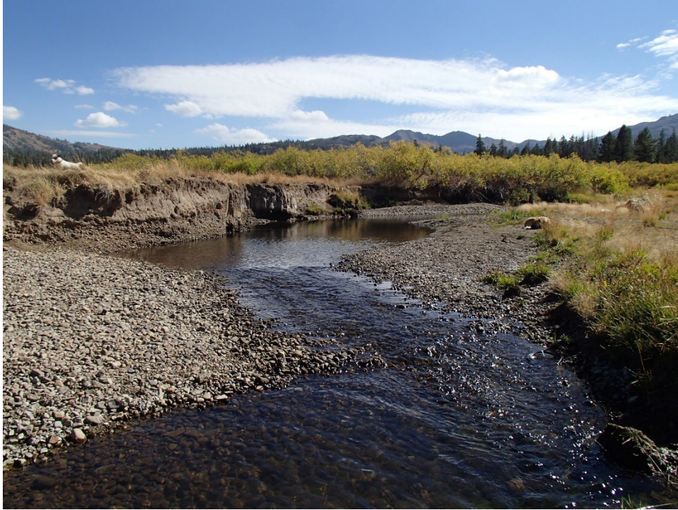
Figure 37. A cutbank still actively eroding. The historic floodplain is still largely disconnected from the stream GM2_2016. Near SSLS17.
