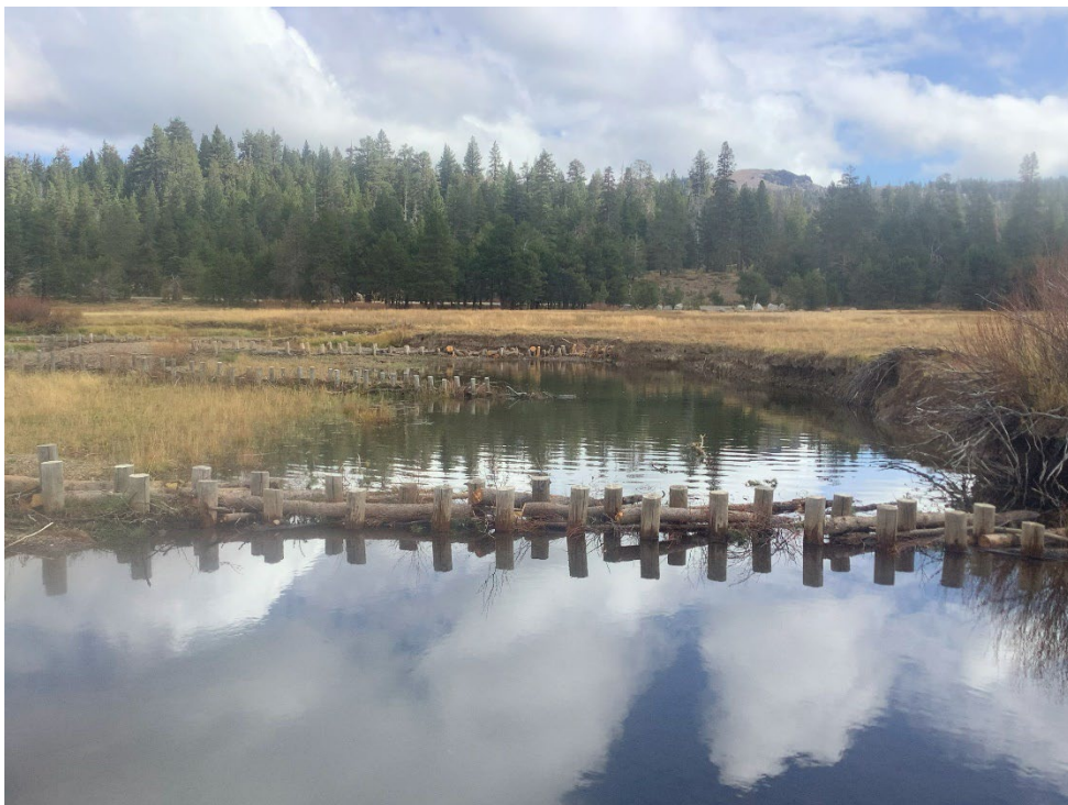
Figure 40. The same section of channel as in Figure 35 post-treatment. A complex of structures drives sediment deposition, a higher water table, deeper pools, and slower velocities. Emergent vegetation is beginning to take hold on the left bank gravel bar. Note the partial span of the middle structure which was breached in 2023. It continues to do work in the channel despite being breached. GM_2024, SDBV17
