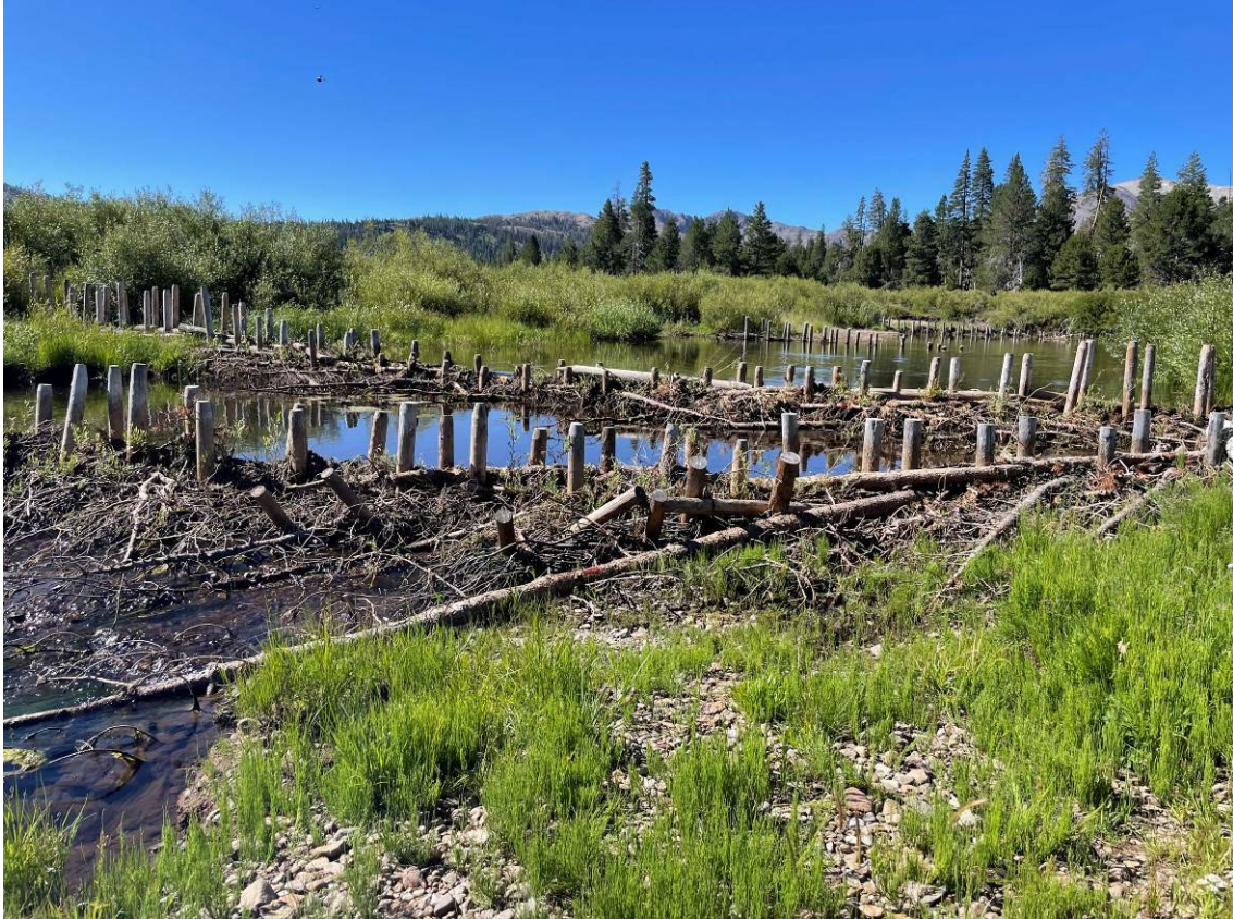
Above: Recently constructed beaver dam analog structures at Faith Valley, Photo by H. Loffland
