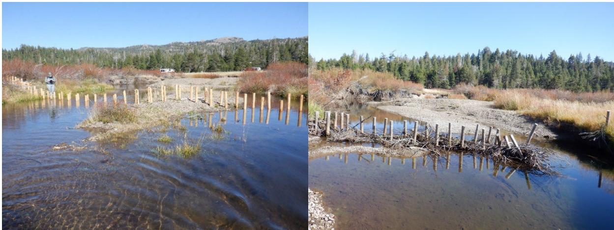
Photo 6. Examples of a partially built BDA (left) where willow weave was not completed (fall 2022) and a blown out BDA (right) in fall 2023.
