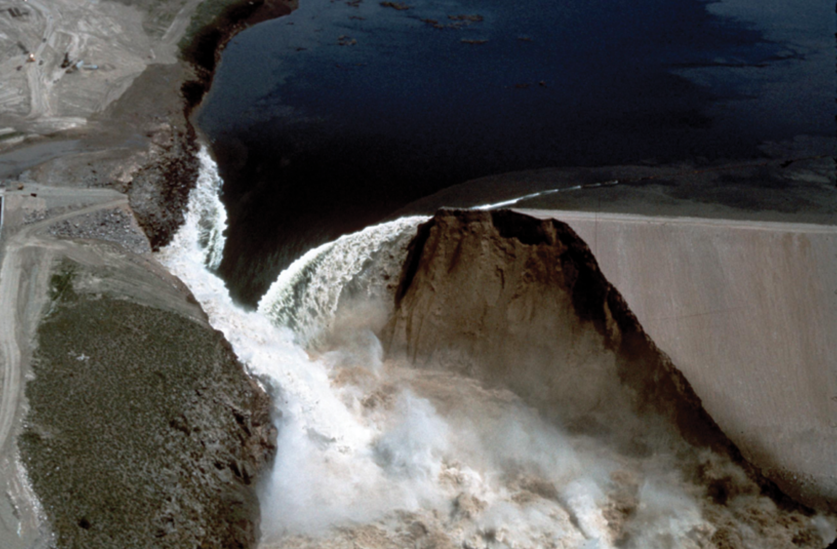
TETON DAM FAILURE. JUNE 5, 1976 SOURCE: WWW.WATERARCHIVES.ORG
