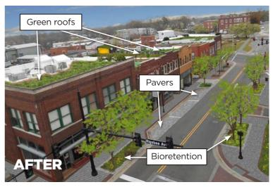
**A Green Street** is a collection of green infrastructure implemented in the street's right-of-way. Green streets incorporate bioretention and permeable pavers in a series to multiply the beneficial impacts.
