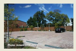
**Permeable paving** includes a range of materials that allow stormwater to move through a "paved" surface. Permeable pavers can be used in residential or commercial settings and are aesthetically comparable or superior to concrete, asphalt, and other impermeable surfaces.
