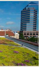
**Green Roofs** store and treat stormwater that falls on rooftops. A greenroof consists of a layer of vegetation and soil installed on top of an existing roof. In addition to reducing stormwater flows and nutrients, green roofs may also: reduce roofing maintenance, improve building energy efficiency, reduce urban heat island, provide habitat for wildlife, and improve air quality.
