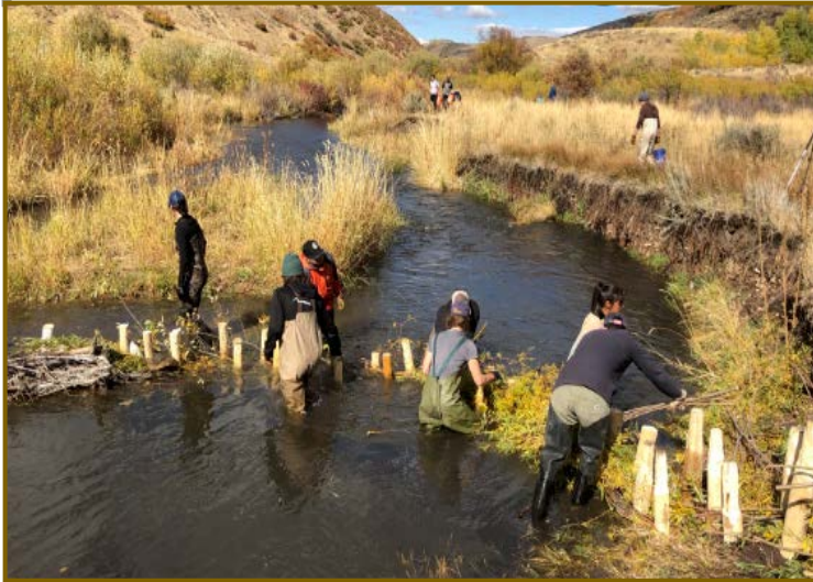
BDA project in East Canyon Creek, Utah, Photo by Mark Edgley
