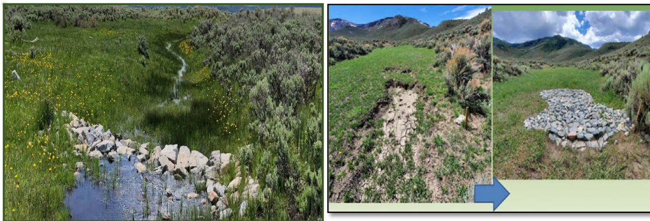
Photos by Shawn Conner, Bio-Logic, Inc., of LTPBR projects he worked on with many partners that used Zeedyk rock structures to restore rangeland mesic areas in the Upper Gunnison Basin.
