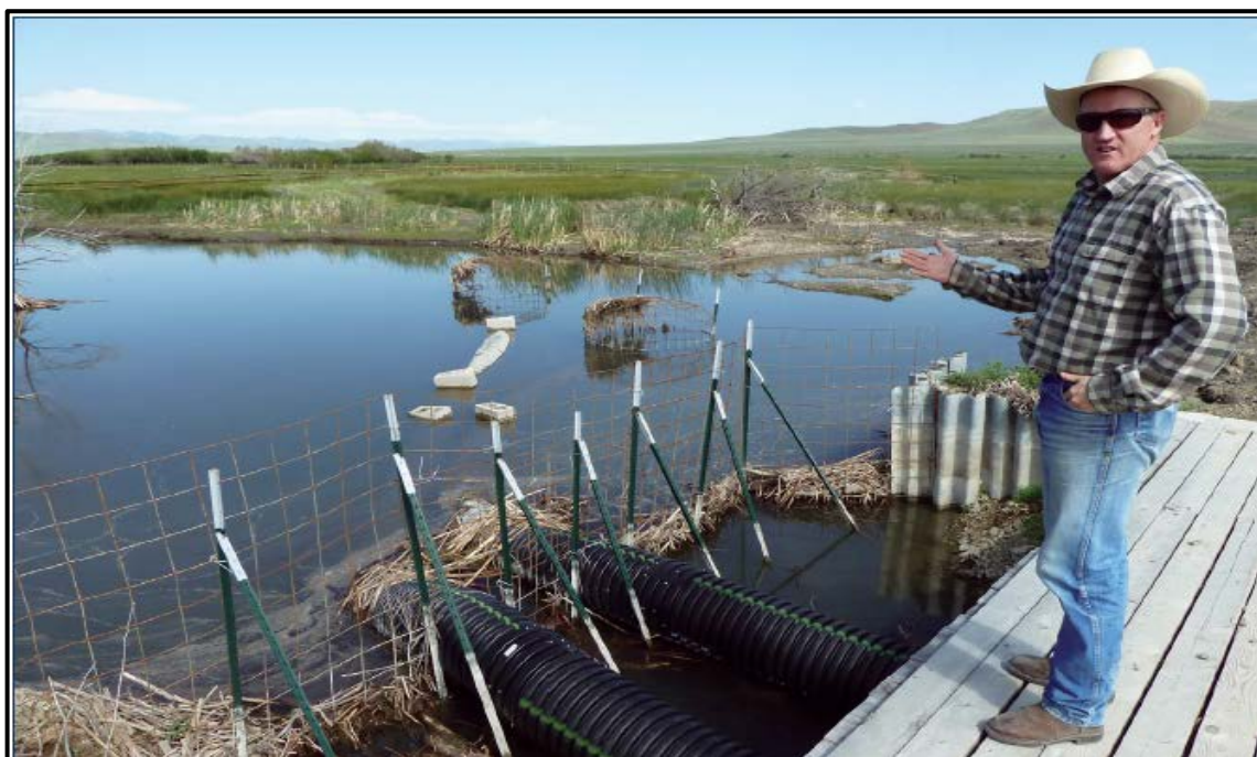
Photo by Dr. Susan Charnley showing a method to stop beaver flooding of a ranch road culvert.
