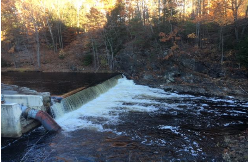
Photo 2: Back Dam under normal conditions
