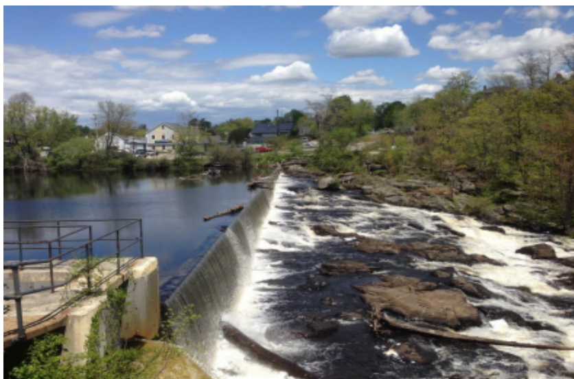
Photo 1: Stone Dam under normal conditions
