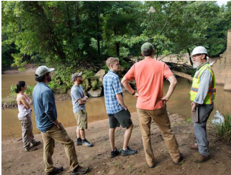
Prior to removal, a viewing zone for visitors should be established a safe distance from the active site
