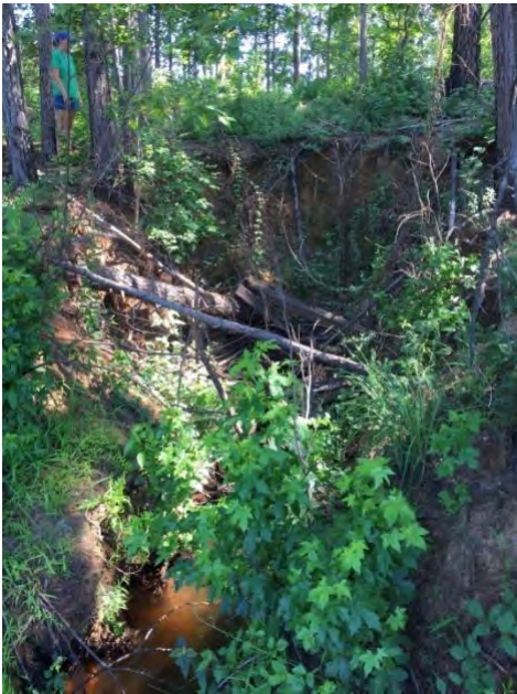
Figure 5: Erosion at Little Pine Knot Dam face
