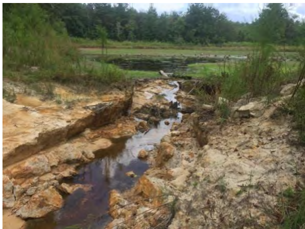
Figure 3: Breach of lowest dam on Hopkins Tract, looking upstream
