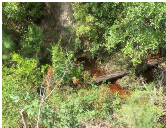
Figure 4: Standing on the top of the breached middle dam looking down (~10 ft tall) on Hopkins Tract
