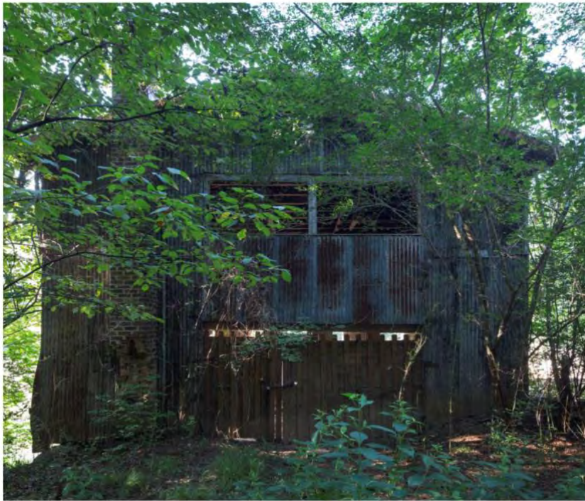
Figure 3: Hydroelectric power plant for the White Dam
