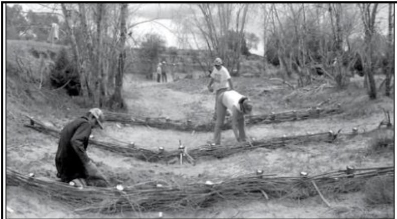
Workshop volunteers build a wicker weir on Largo Creek, Williams Ranch, Quemado, NM. August 2004. Photo by Tamara Gadzia.
