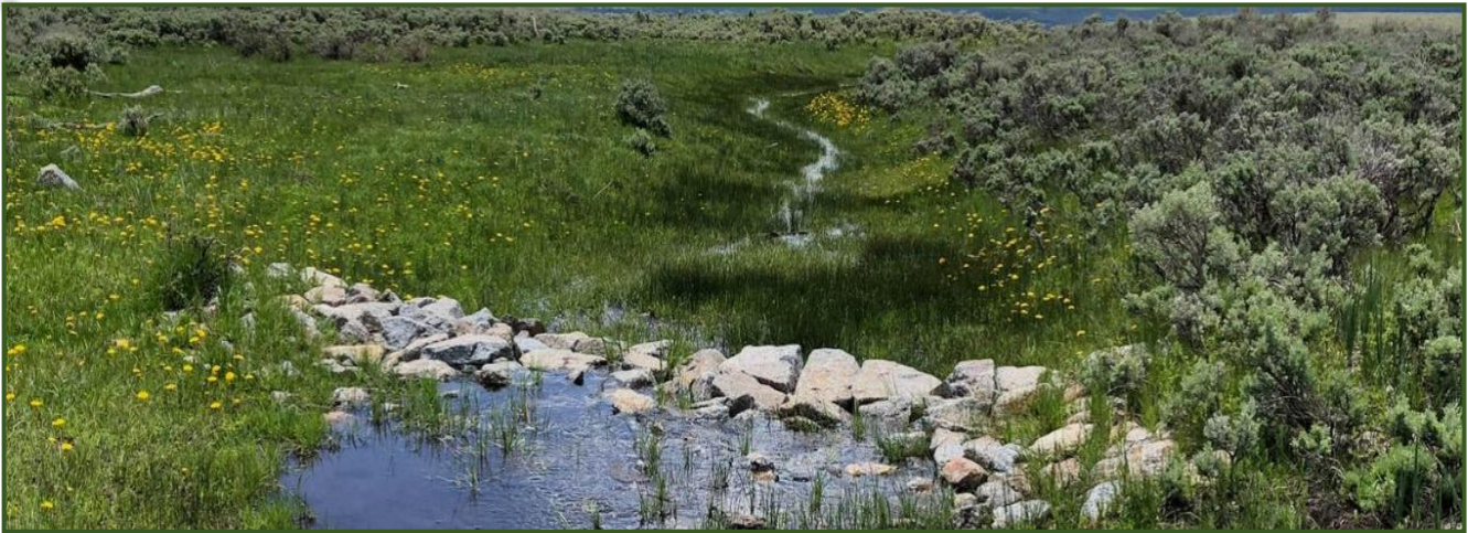
Photo by Shawn Conner, Bio-Logic, Inc., of a LTPBR project that used Zeedyk rock structures to restore a rangeland mesic area in the Upper Gunnison Basin.
