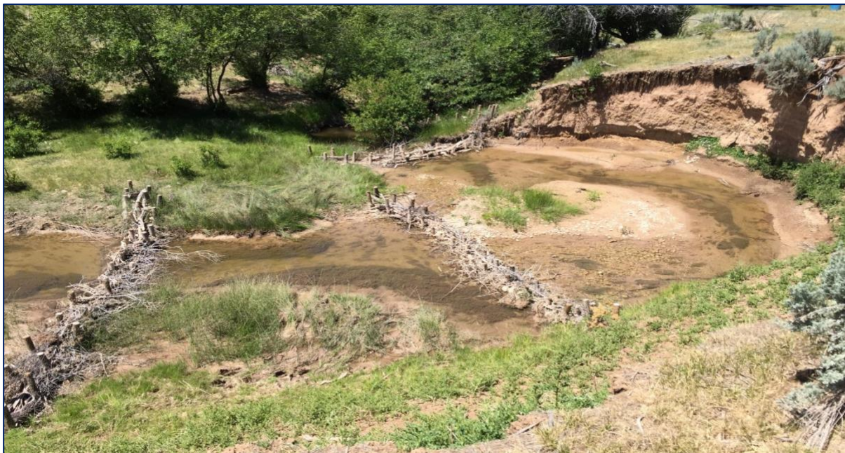
BDA installed in 2019 on Fish Creek on a private ranch near Coalville, Utah; photo by Rose Smith, Sageland Collaborative Stream Ecologist
