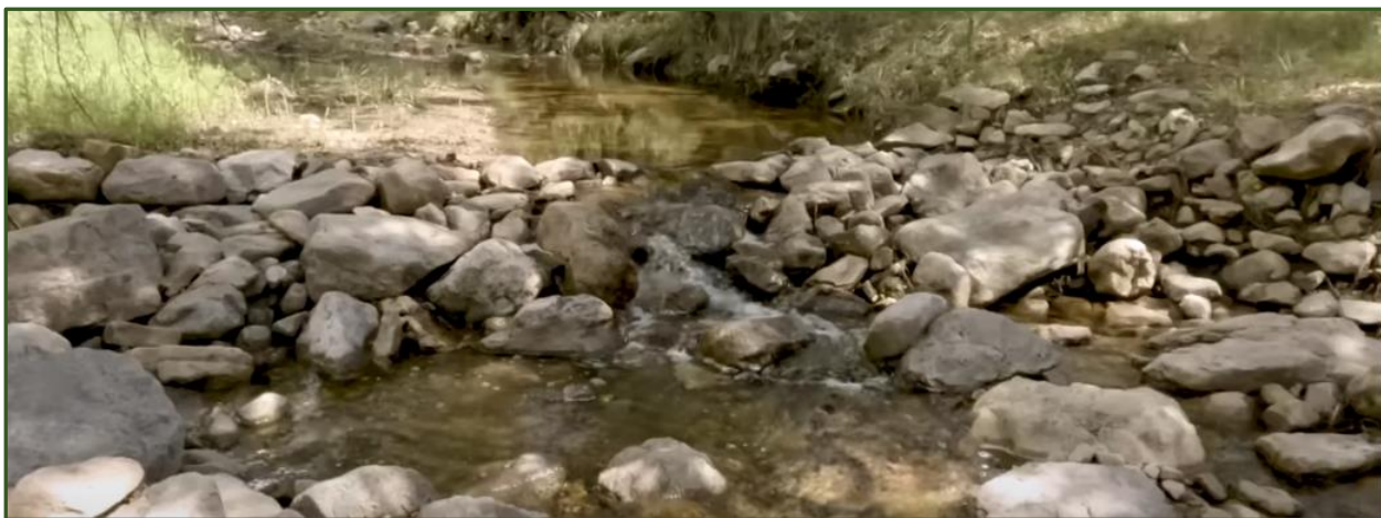
Photo of an example of a rock detention structure on an Arizona creek from the June 2022 video Re-greening a Dryland Watershed | U.S. Geological Survey (usgs.gov) .
