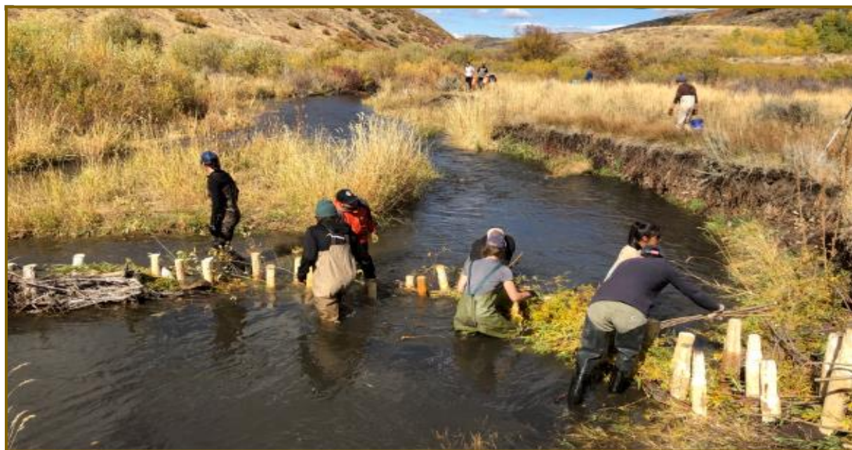
BDAs being installed in East Canyon Creek, Wasatch Mountains area, Utah. Photo by Mark Elzey
