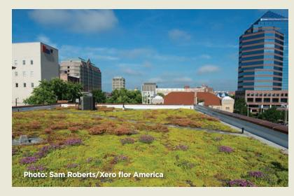
Green Roofs store and treat stormwater that falls on rooftops. A greenroof consists of a layer of vegetation and soil installed on top of an existing roof. In addition to reducing stormwater flows and nutrients, green roofs may also: reduce roofing maintenance, improve building energy efficiency, reduce urban heat island, provide habitat for wildlife, and improve air quality.
