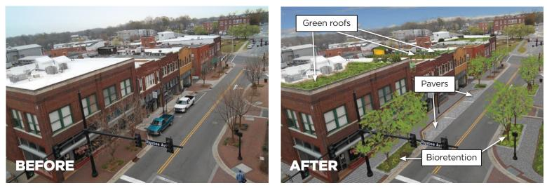
**A Green Street** is a collection of green infrastructure implemented in the street's right-of-way. Green streets incorporate bioretention and permeable pavers in a series to multiply the beneficial impacts.
