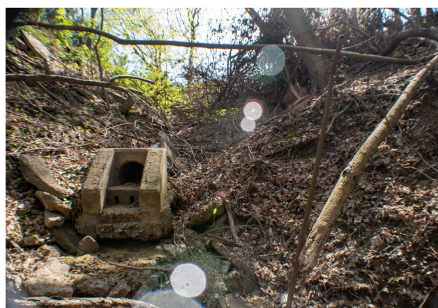
This undersized stormwater outfall broke, causing the collapse of the ground above and around the outfall and displacing the outfall structure about 30 feet away from the rest of pipe, East Moline, Illinois. Photo credit: Olivia Dorothy
