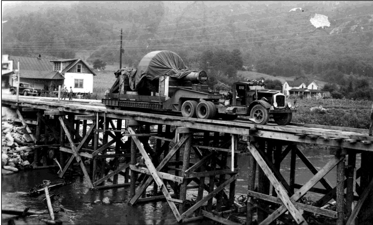
Hydro Unit Crossing Tuckasegee River for Installation in NP&L's (now Duke Energy's) Thorpe Hydro Station – 1941 (photo from Fred Alexander)
