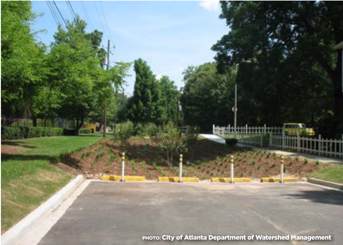
A dead end street retrofitted with a rain garden in the Custer Combined Sewage Area.
