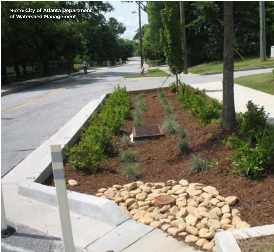
A street bump out using bioretention.
