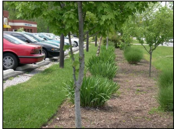
Grass filter strip as a pretreatment to an infiltration area
