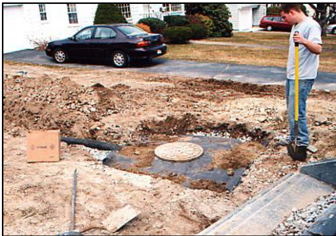
Courtesy of Nicholls Landscaping Residential dry well for roof runoff and sump pump drainage
