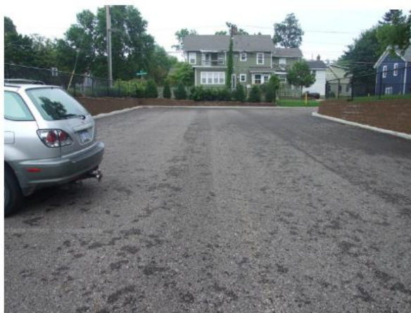
Porous asphalt parking lot
