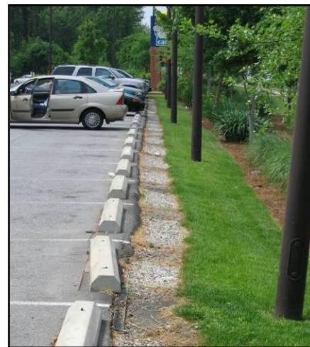
Gravel diaphragm upstream of grass filter
