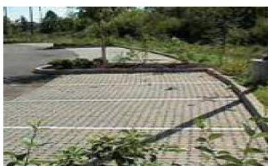
Permeable paver block parking lane
