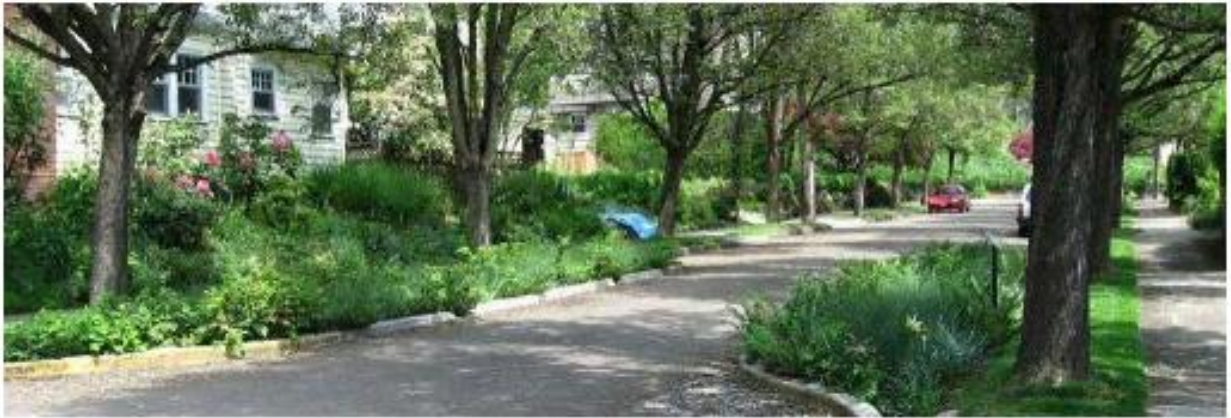
Curb Extension Bioretention
