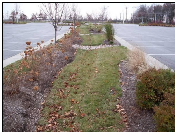
Bioswale at The Shops at Fallen Timbers in Maumee, Ohio
