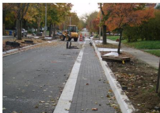
Permeable paver block parking lane
