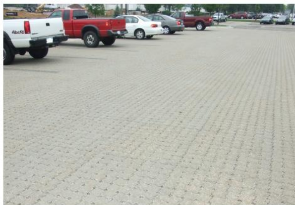
Permeable paver block parking lot
