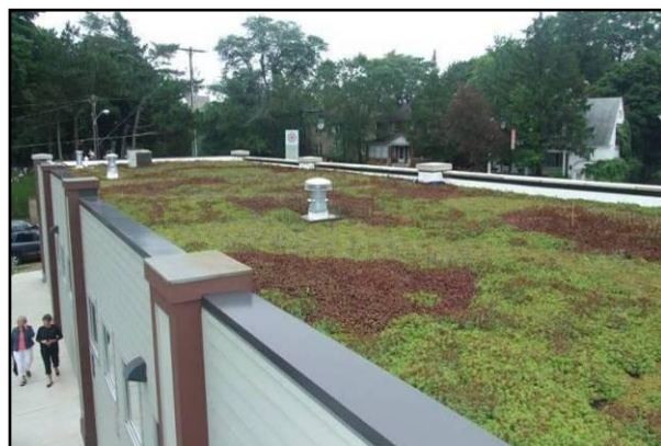
Extensive vegetated roof planted with sedum on a commercial building
