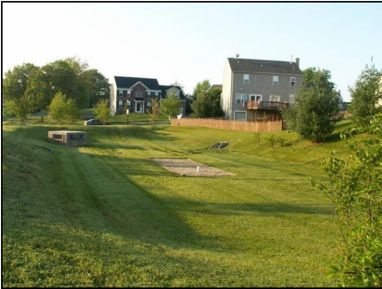
Courtesy of Montgomery County, Maryland Pocket sand filter in a residential area
