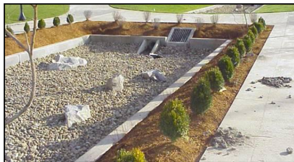
Courtesy of City of Portland, Oregon Pocket sand filter
