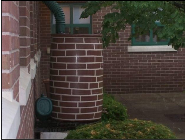
Rain barrel collecting roof runoff at a municipal building
