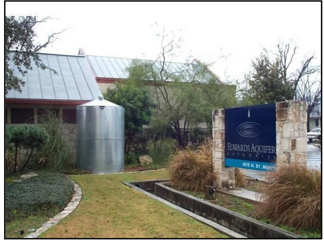
Courtesy of The Texas Water Development Board Cistern collecting roof runoff at a commercial building
