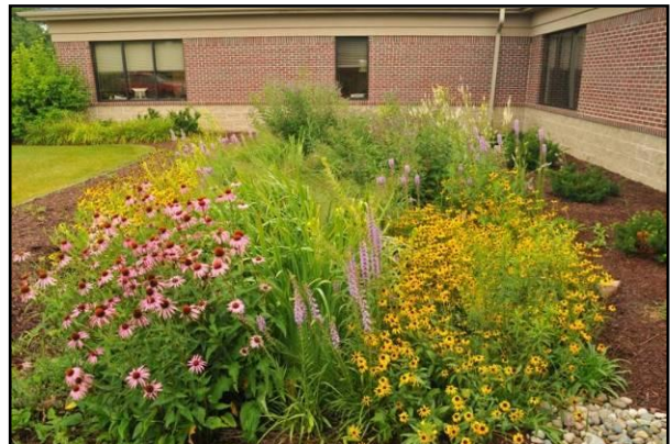
Bioretention at an office building
