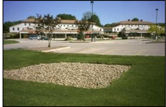
Courtesy of Wisconsin Department of Natural Resources Infiltration trench with grass filter strip adjacent to parking lot
