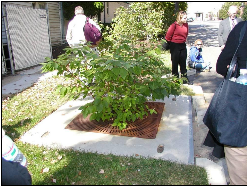
Courtesy of Larry Coffman Tree box along local street
