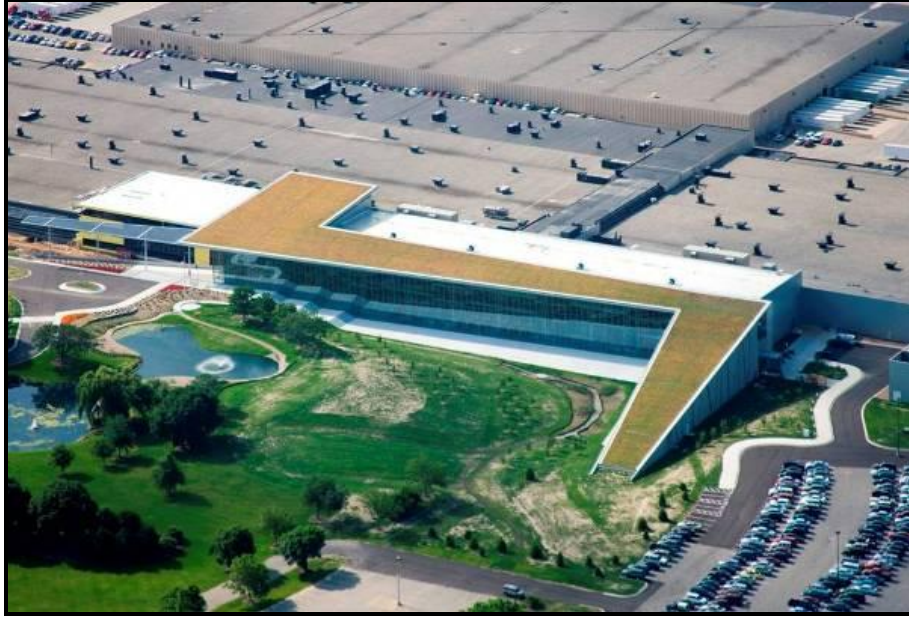
Courtesy of Haworth Corporation Grand Rapids, Michigan Vegetated roof on a commercial building
