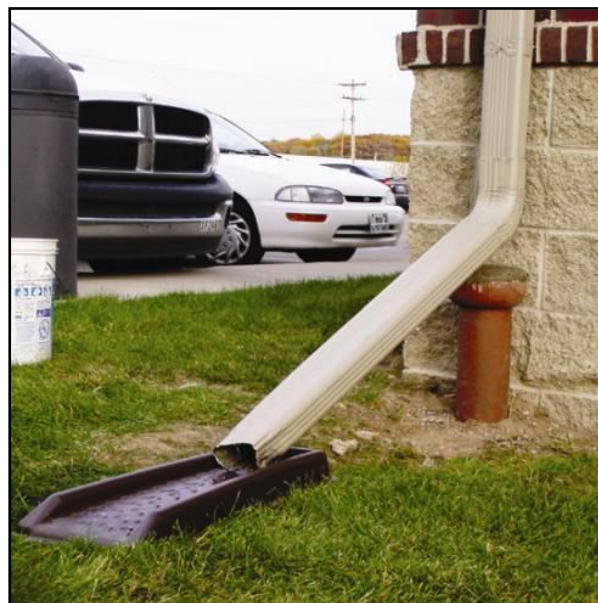
Disconnected downspout
