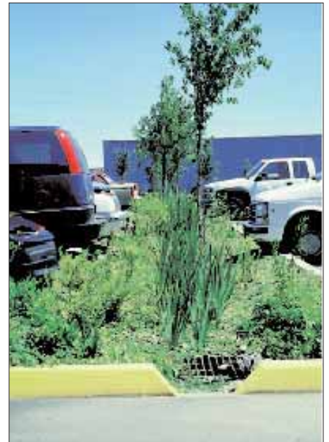
Parking median bioretention with curb cut (Photo: Portland Bureau of Environmental Service)
