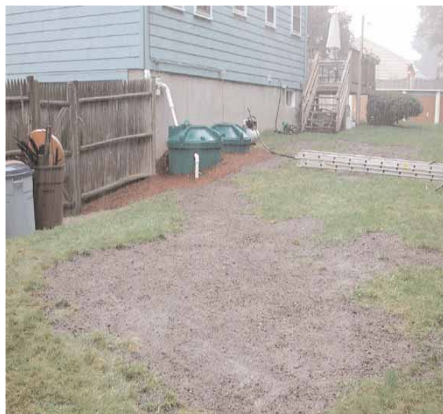
Manufactured dry well system after installation. The dirt areas indicate where the well was buried. The green objects are storage tanks with a pump. Drywells also work well receiving rain barrel overflow (Photo: Charles River Watershed Association)
