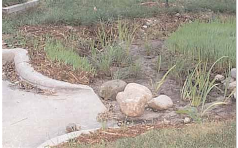
A curb cut into a small bioretention area (Photo: Applied Ecological Service, Inc.)
