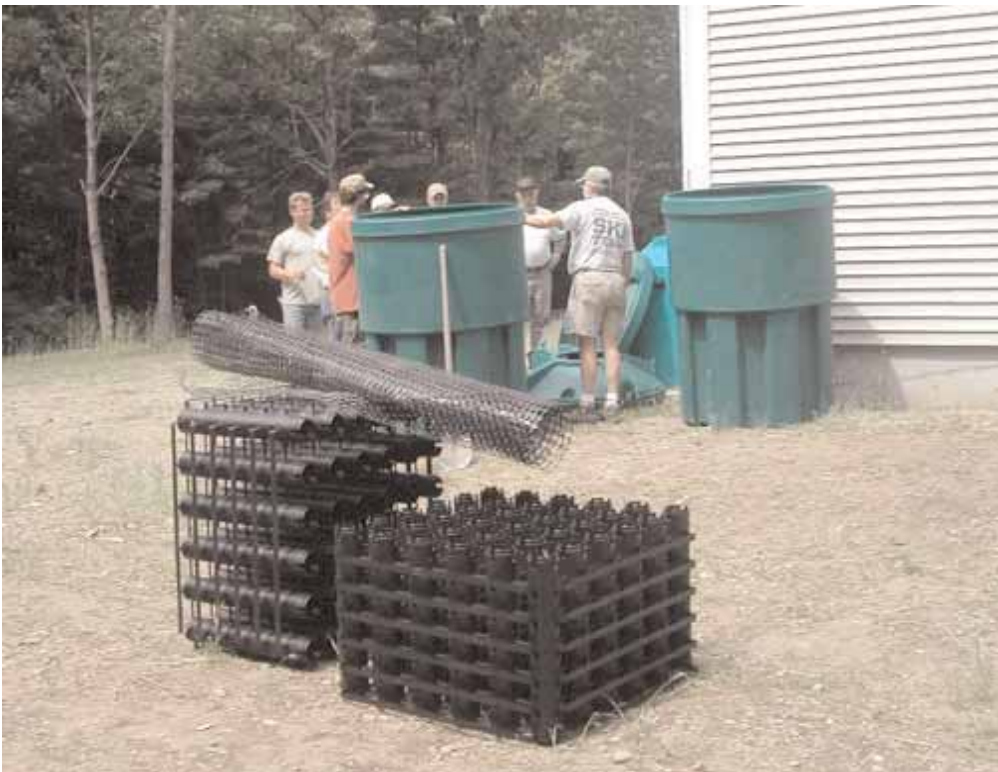
The black grids are part of a manufactured dry well. Once installed in the ground, stormwater will be funneled to storage in the grid system (Photo: Charles River Watershed Association)
