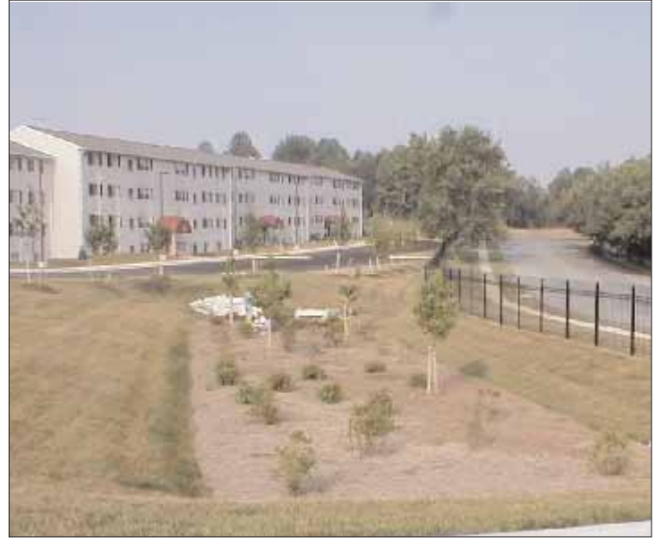
An infiltration basin using bioretention in Largo, Maryland (Photo: Dr. Allen Davis, University of Maryland)
