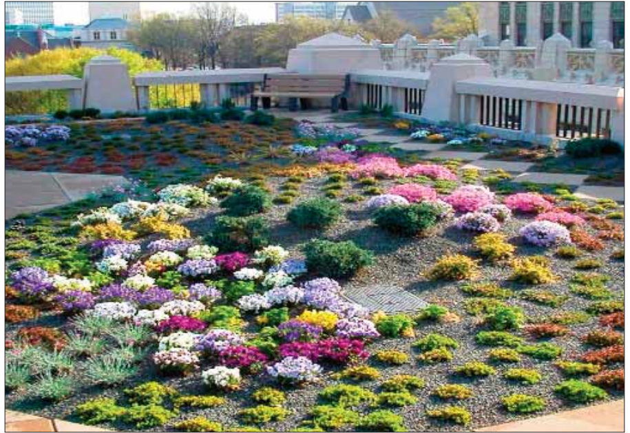
The green roof atop Atlanta's City Hall (Photo: City of Atlanta)
