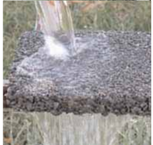
The top photo is of grass pavers. If grass is undesired, gravel or stones can also be used. The lower photo is of pervious pavement (Top Photo: Todd Litman, VTPI; Bottom Photo: John Cummins, PermaPave)
