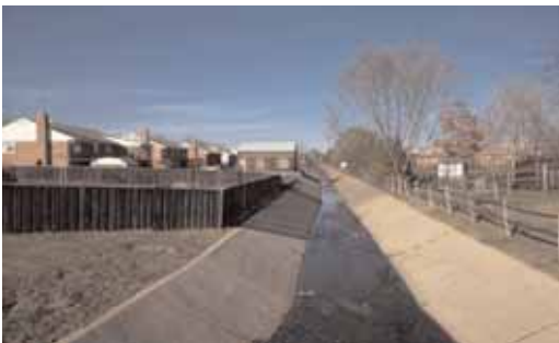
A channelized stream in a suburban neighborhood (Photo: United States Department of Agriculture)
