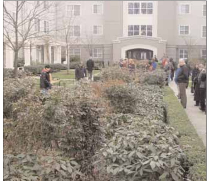
A bioretention area in an apartment complex in Portland, Oregon (Photo: Betsy Otto)
